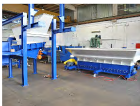
Crusher & Scraps treatment
